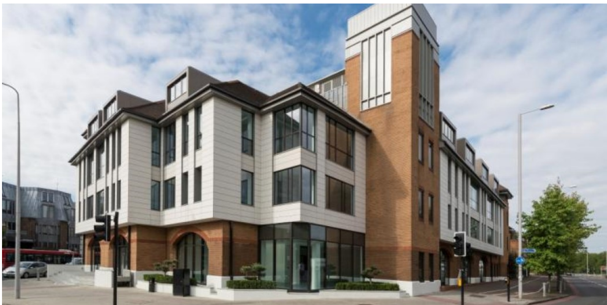
Following our refurbishments which included an upgraded façade, full M&E replacement and car parking spaces removed in favour of cycle bays, this building in Richmond London fetched an ungeared IRR of close to 52.4% over a period of 16 months 4 . For illustrative purposes only.
